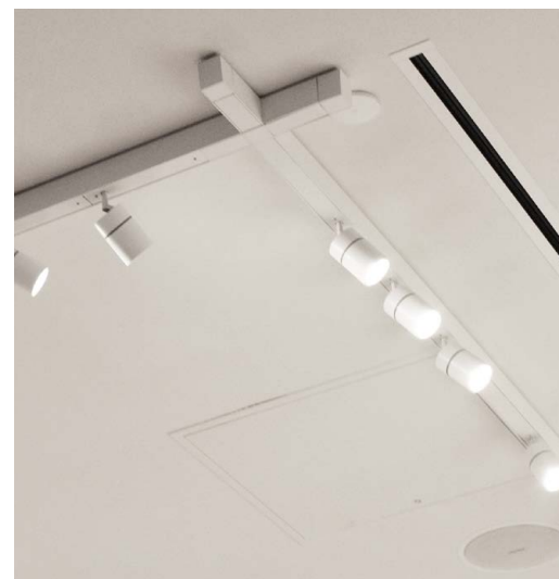
FIXED CEILING W. ACCESSIBLE INSTALLATIONS
