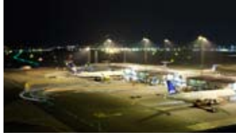
Energy consumption at Copenhagen Airport is highest in the terminal areas. The focus on energy conservation is therefore especially concentrated on that area.
